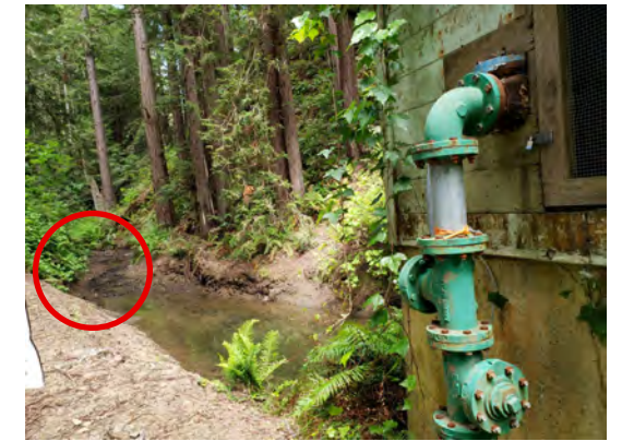
Sample Site No. 2-b Pumping Station
