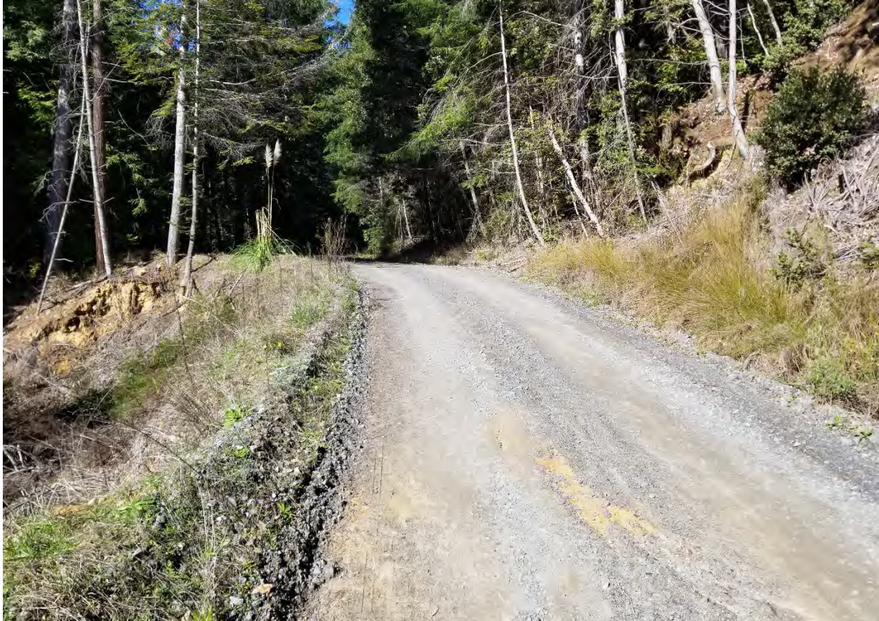
Figure 5.3.4-1 Plant Unpaved Access Road and Wash-Out Area
