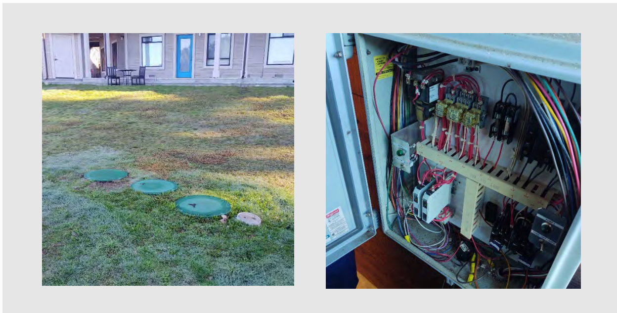
Figure 2.4.1-1 Commercial Septic Tank Lids and Panel
