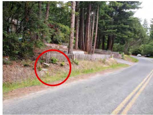
Sample Site No. 1 Pipe Outlet
