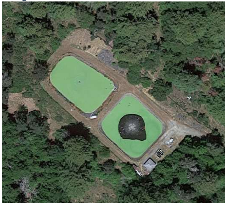
Figure 3-2: Aerial View of Wastewater Treatment Plant
